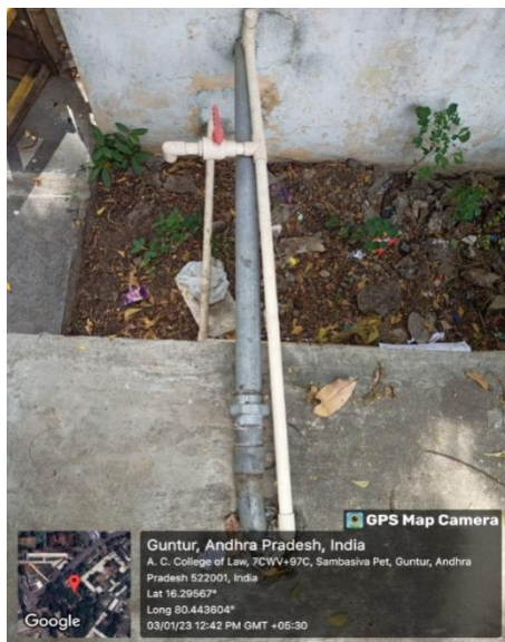
Fig 3: Waste water from RO plant is used to recharge open bore well
